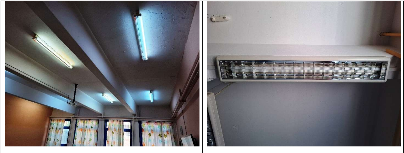
Figure 13: Existing luminaires
