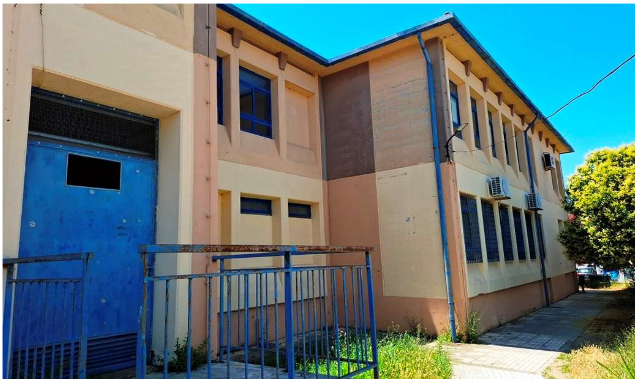
Figure 12: Part of the North façade of the building
