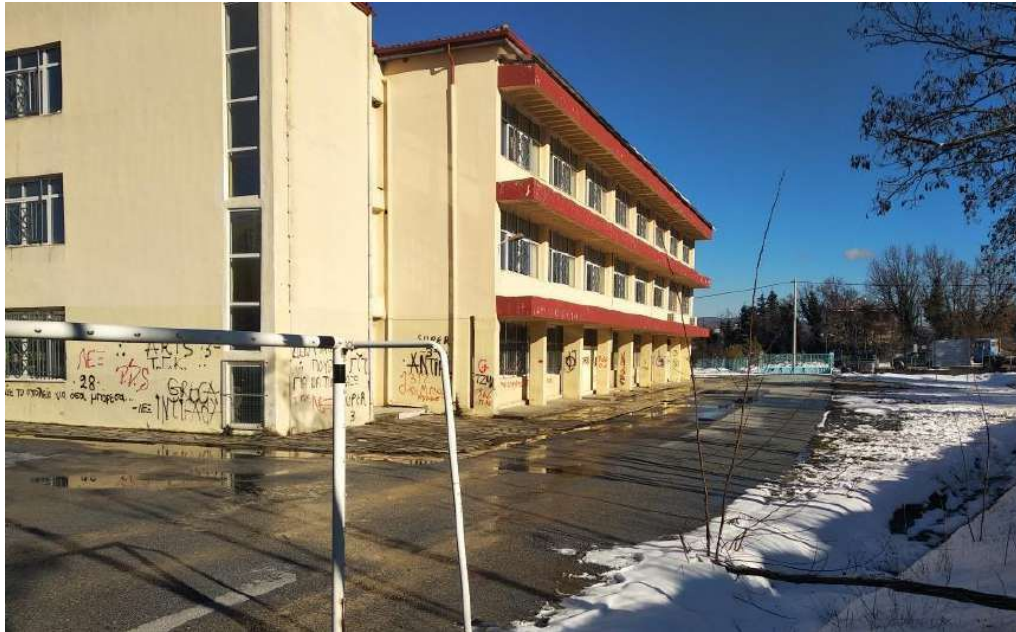
Figure 4: Part of the North and West façade of the building
